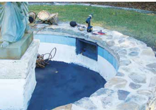
Relining and laying stone for the fountain featuring Mary and the Blessed Child
