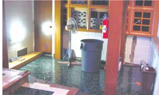
The new floor installed for the choir loft at St. Mary on the Hill
